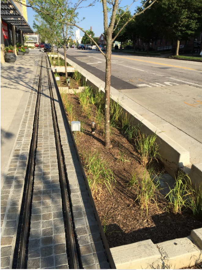
Figure 4.5. Example streetscape bioretention.
